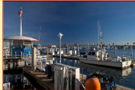
Marine Fuel Facilities
